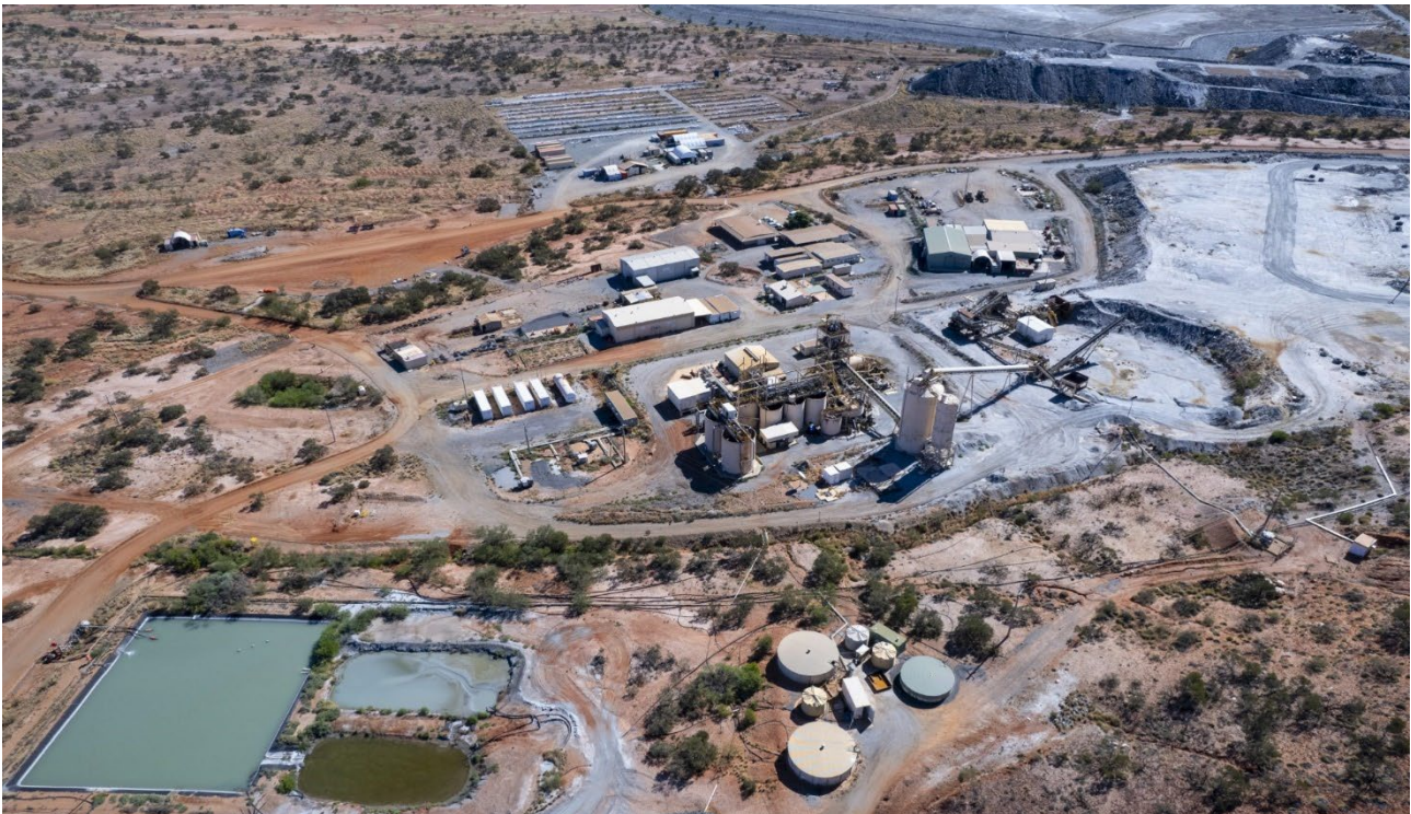
Figure 2: July 2023 drone photograph of the Paulsens 450ktpa processing facility and other infrastructure
