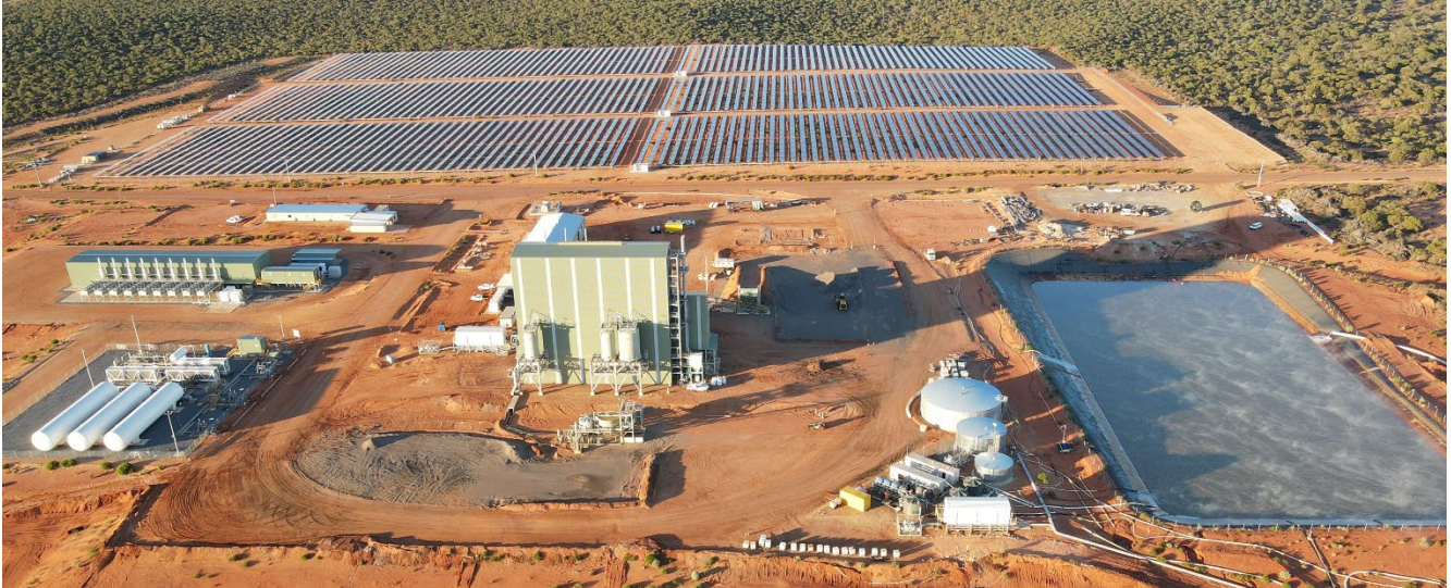
Figure 1 Coburn Project - Mineral Separation Plant
