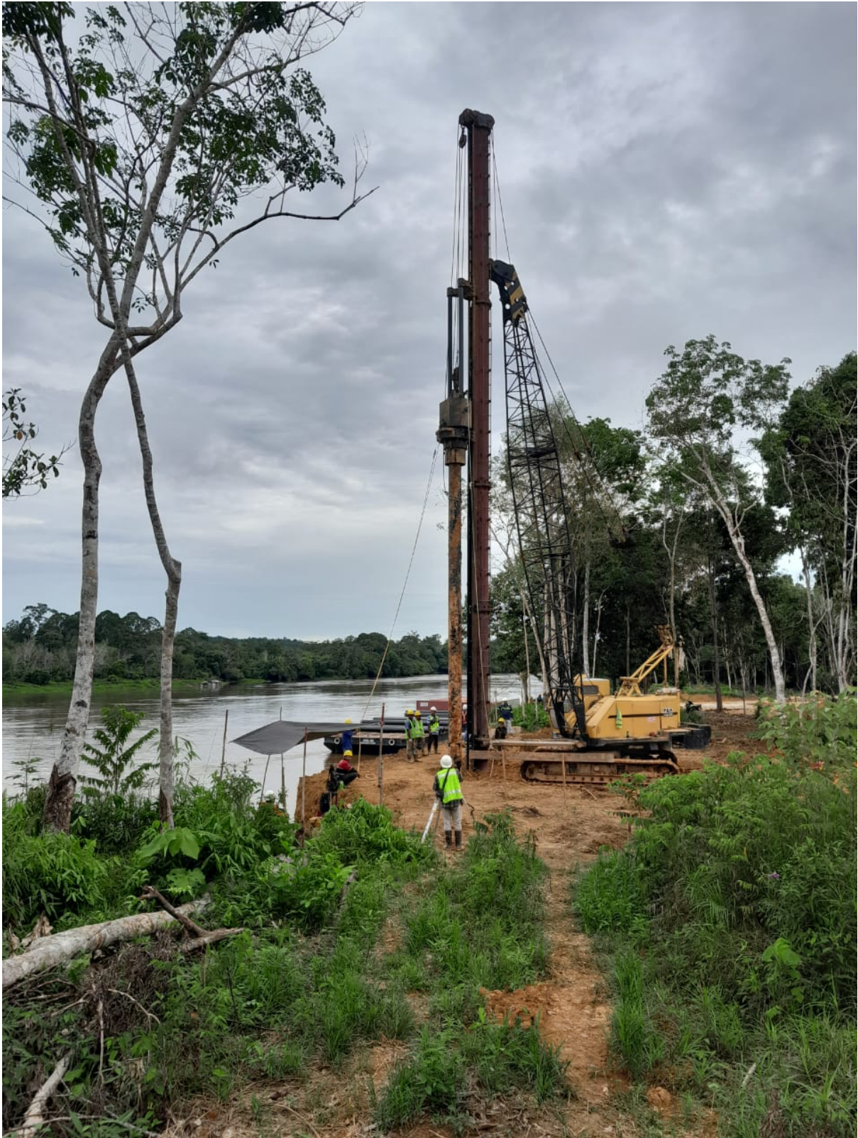
Piling Works at Jetty
