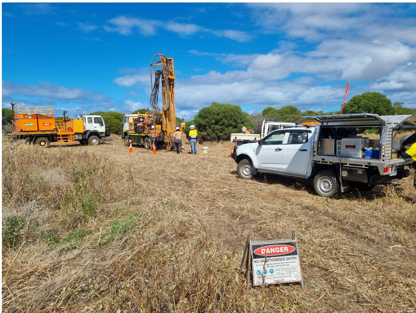
Figure 5: Bostech drilling rig on site
