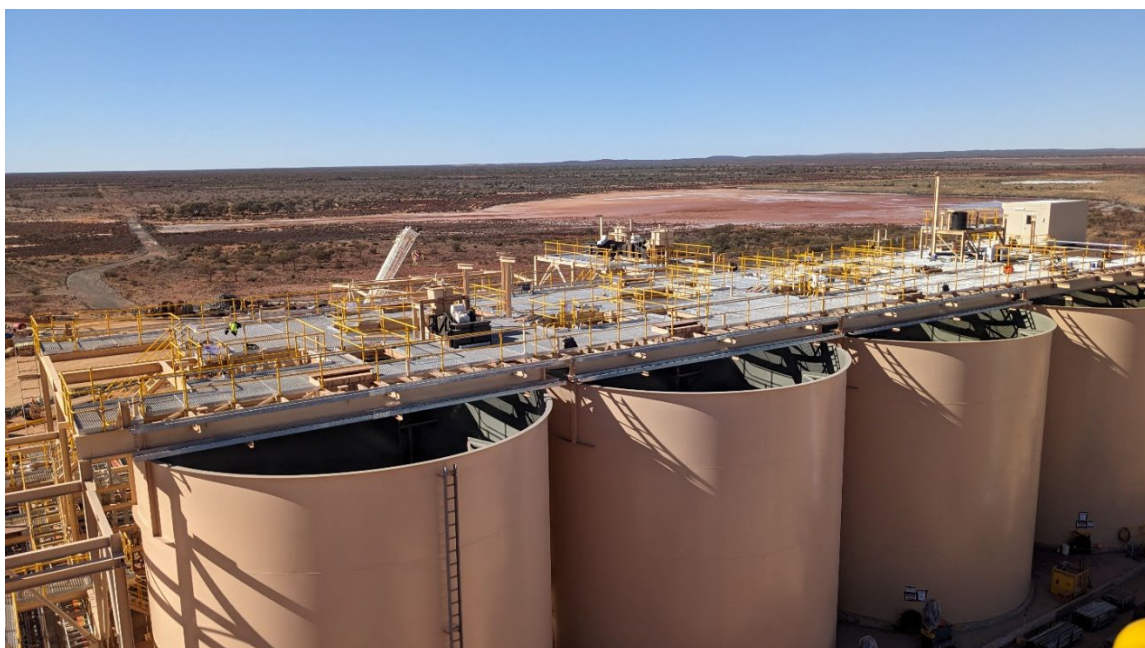
Figure 3: CIL top of tank steel works completed.
