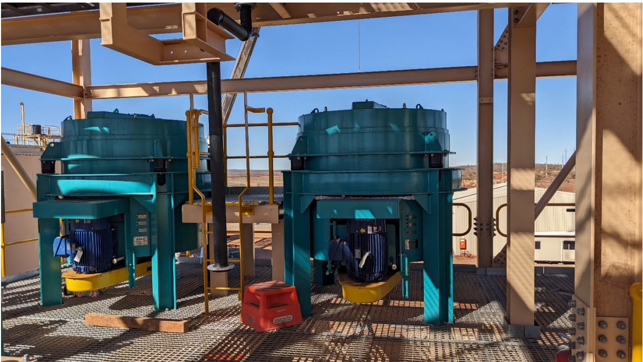
Figure 5: Installation of the Knelson concentrators.
