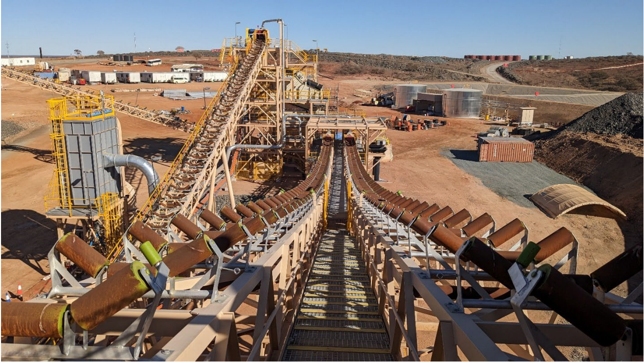
Figure 4: Completion of conveyor structures with belt installation to commence next week.
