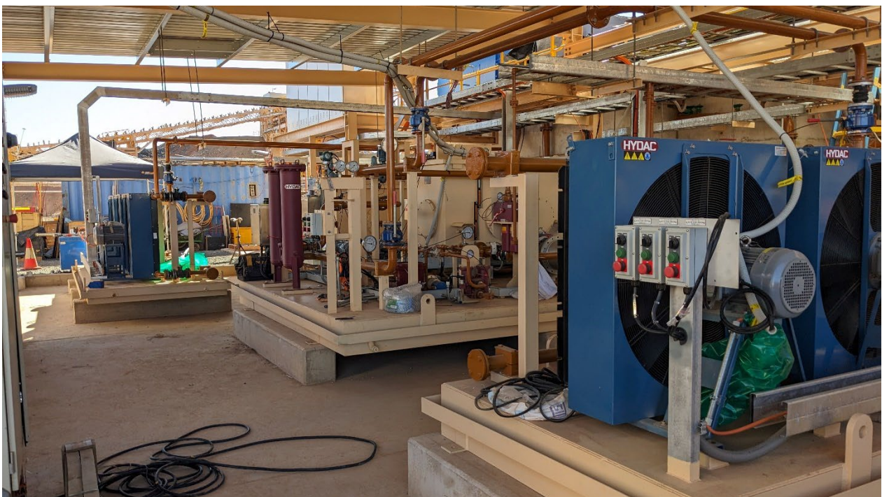
Figure 7: Mill lube station installation.
