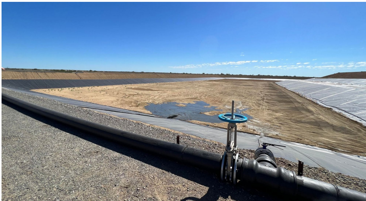
Photo 2. First tailings being deposited into the newly commissioned TD5.
