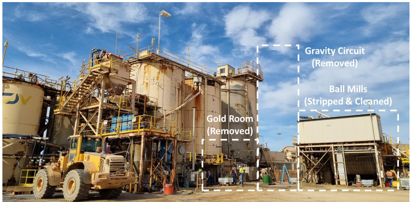
Figure 3 – Central Gawler Mill with gravity circuit, gold room and other key equipment removed 2
