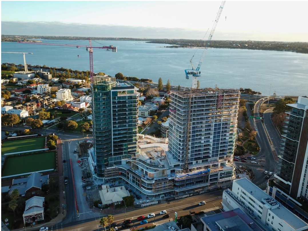
ABOVE: View to West showing Mends Street tower (left of picture) completed, and Mill Point Tower structure (right of picture) reaching level 21 of 38.
