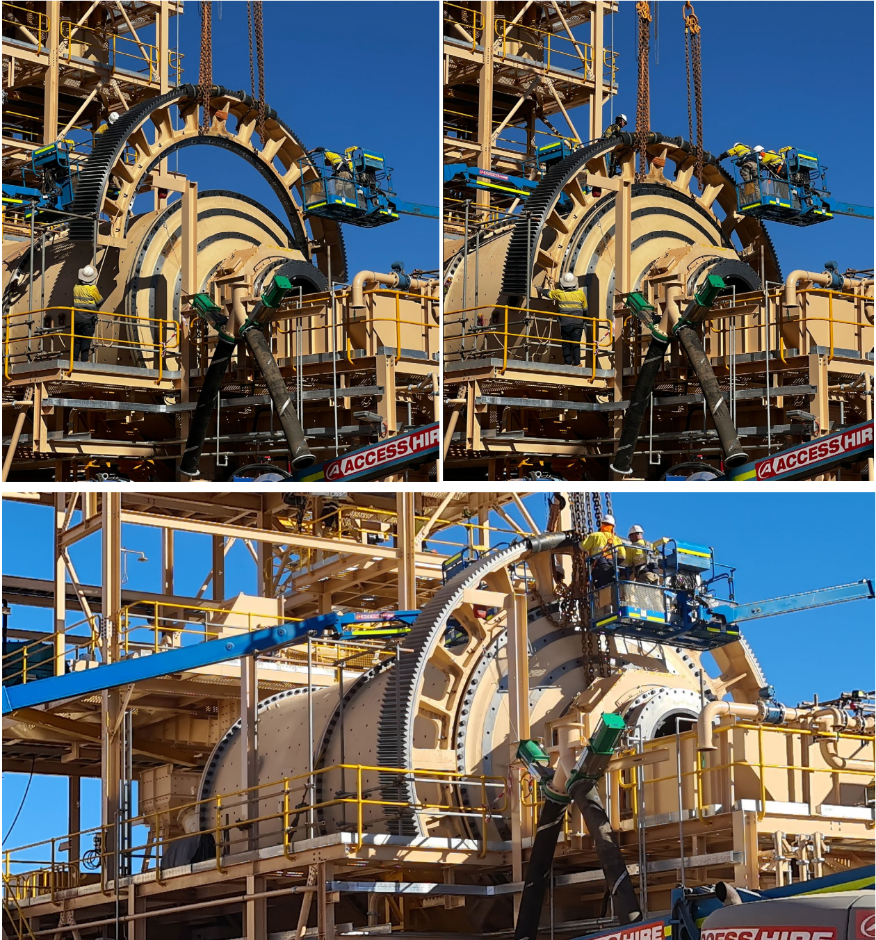
Figure 2-4: Ball mill girth gear installed in July 2023.
