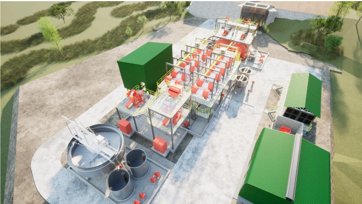
Image 5: Elevated view of the recovery circuit and tails thickener.
