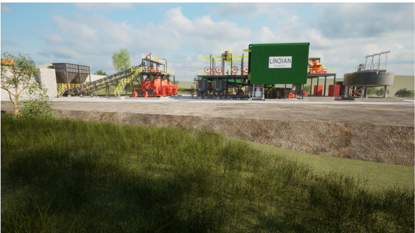
Image 3: Preliminary schematic of plant design from ground level. Existing retaining wall (left), ball mills (centre left), recovery circuit (centre) and tailings thickener (right)
