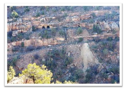
Figure 3. Photo of three mine portals in the upper sandstone layers of the Salt Wash member at the 45-90 mine (see figure 2, above, for location of 45-90)
