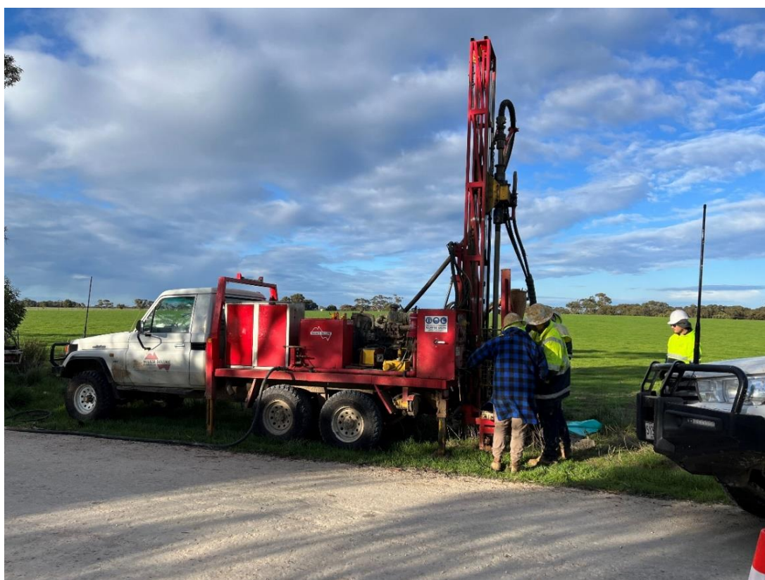
Figure 5: Roadside Drilling Team on Raitz Road north of Bordertown
