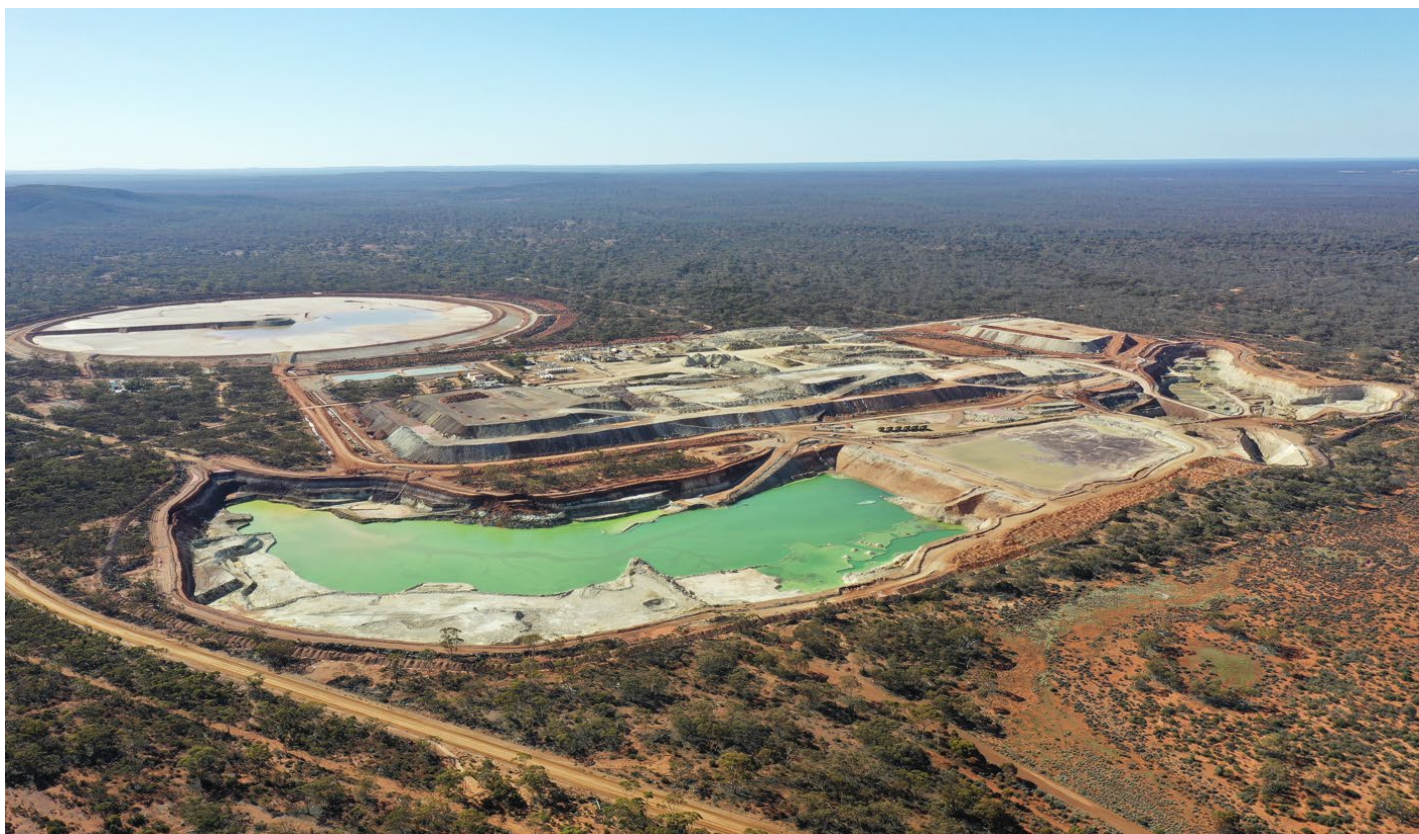
Figure 1: Jaurdi Gold Project on 20 July 2023
