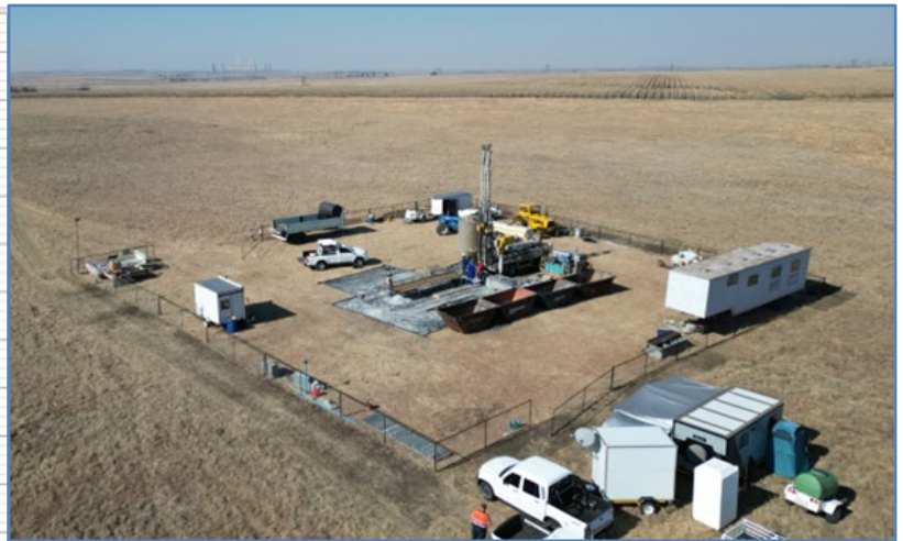
Figure 8 - Location of 272-06C with Sasol's Secunda plant in the background
