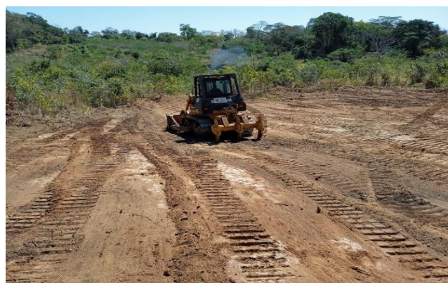
Clearing of regrowth at proposed water dam
