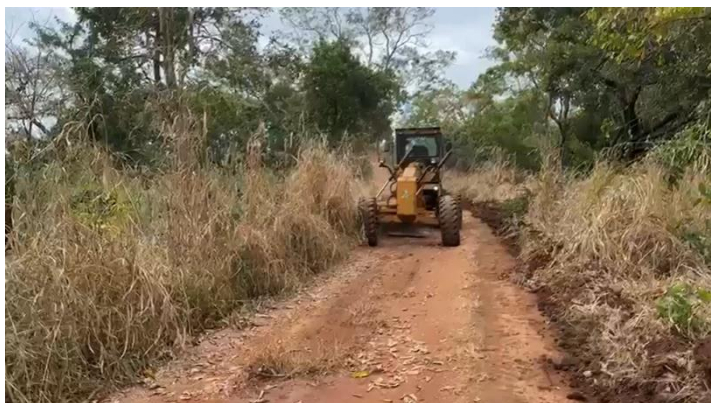
Grading of the Ancuabe main access road
