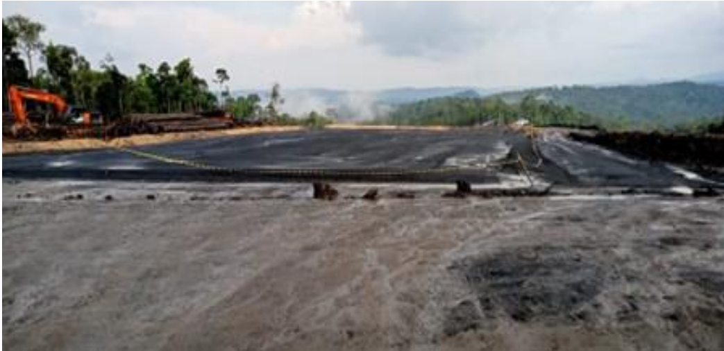
Expansion of ROM Stockpile
