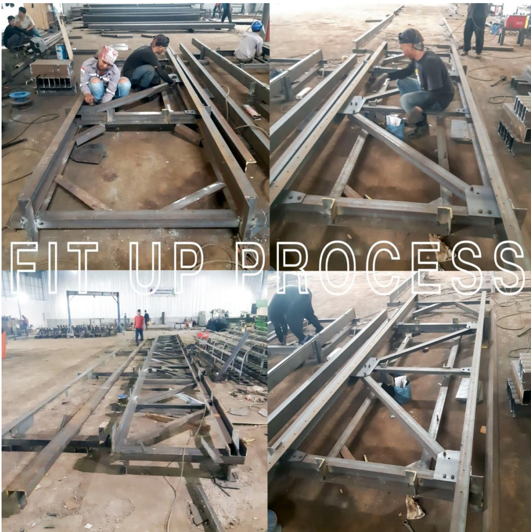
Fabrication Works Progress
