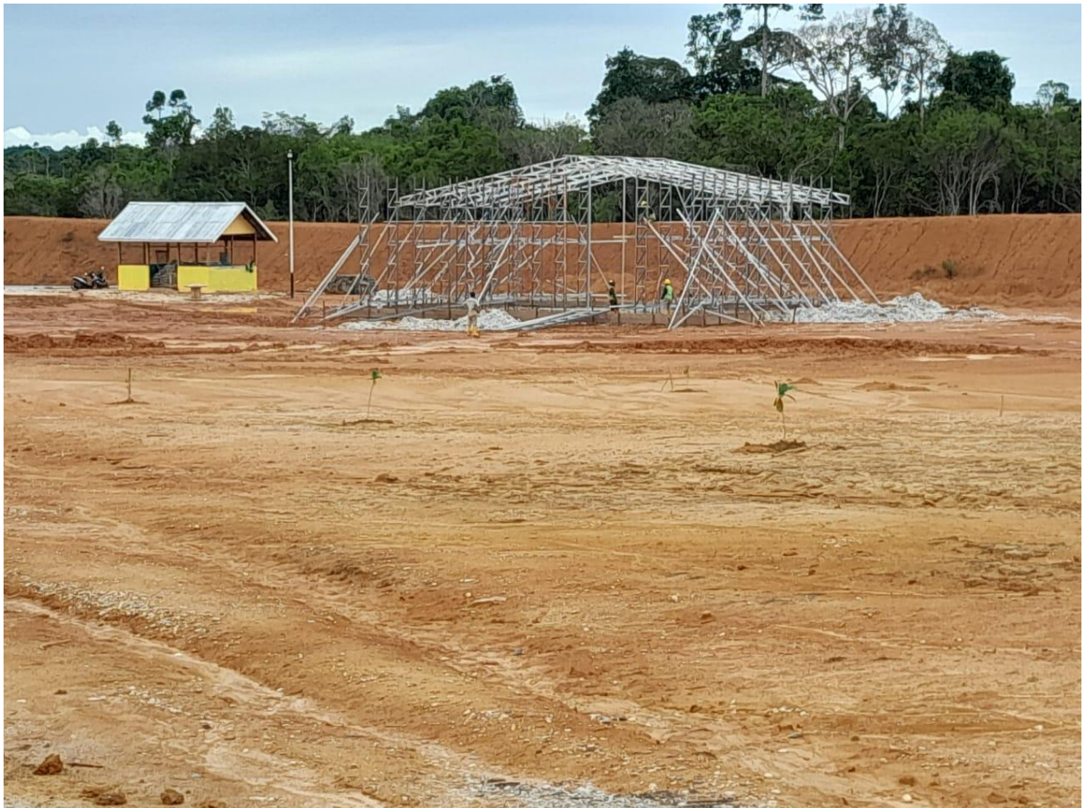
Truck Workshop Construction Progress
