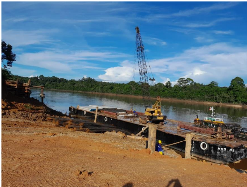
Mobile Crane arrives at Batu Tuhup Jetty
