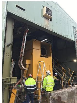
Figure 2. New SAG discharge hopper
