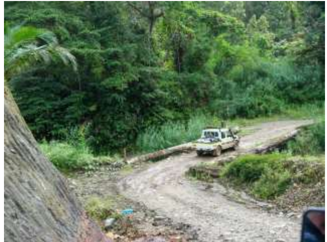
Road network including creek crossings
