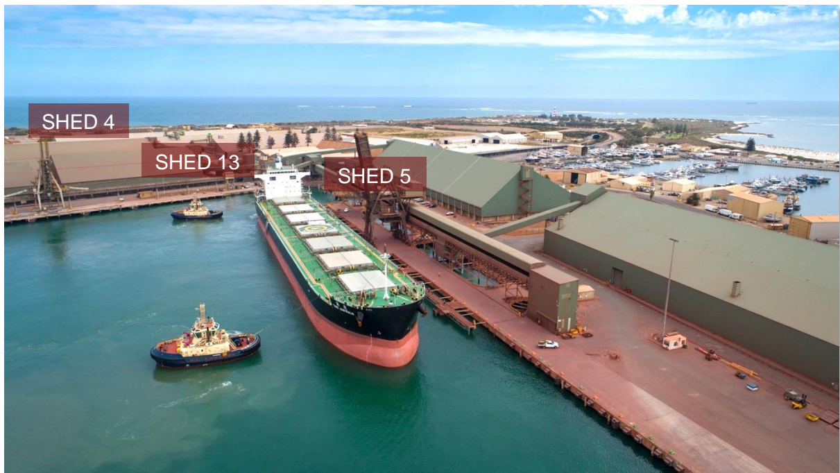
Fenix's Geraldton Port infrastructure
