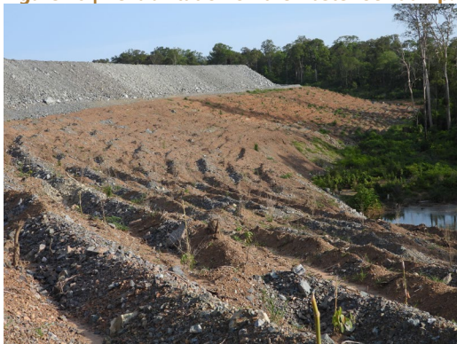
Figure 10 | Rehabilitation on the waste rock dump. Okvau has only one oxide batter
