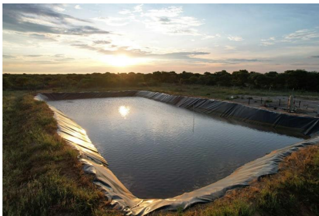
Figure 1 - Serowe 3 Flow testing evaporation pond
