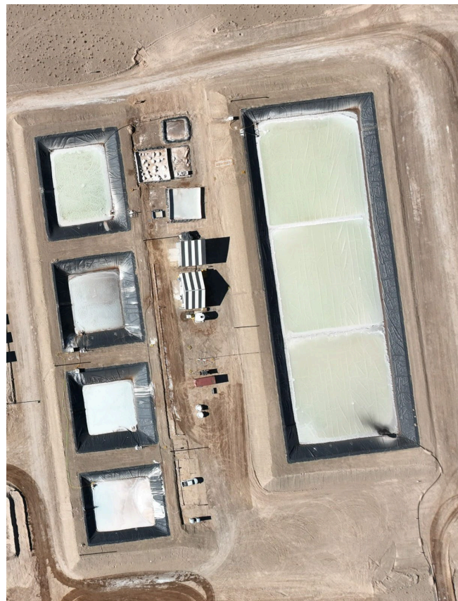
Figure 12: Aerial view of existing pilot plant
