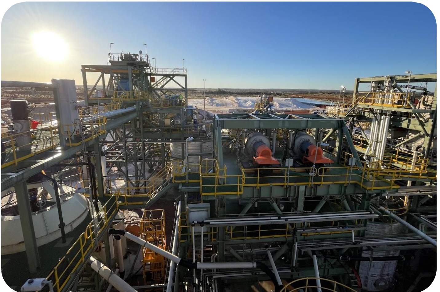
Beyondie SOP plant, June 2023
