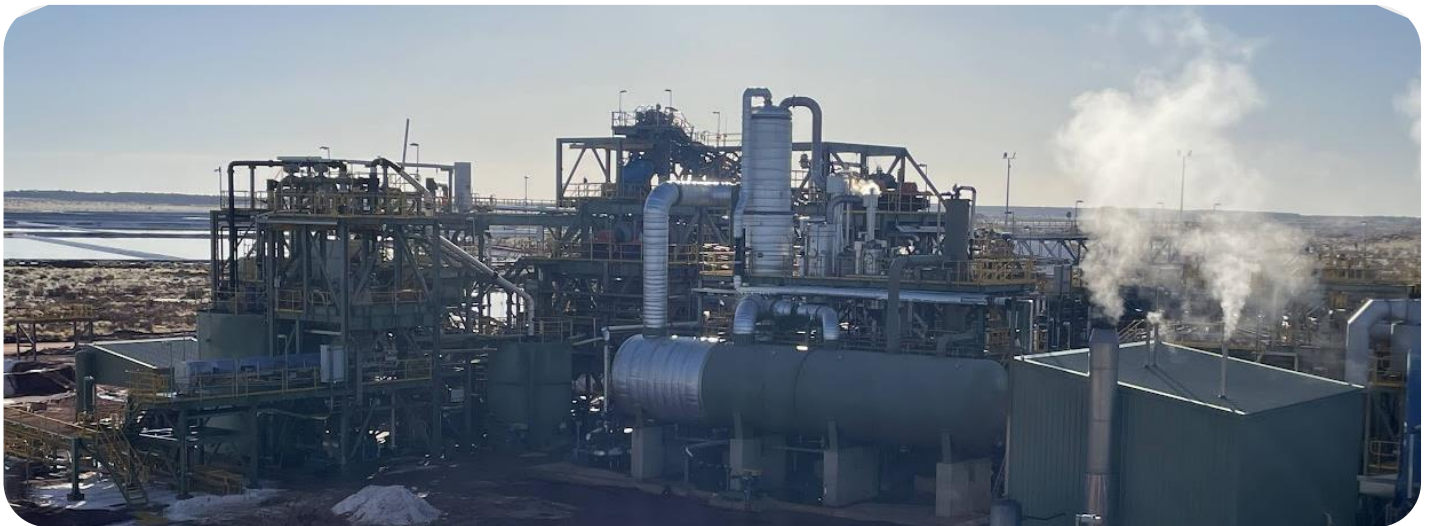
Beyondie SOP Plant, June 2023
