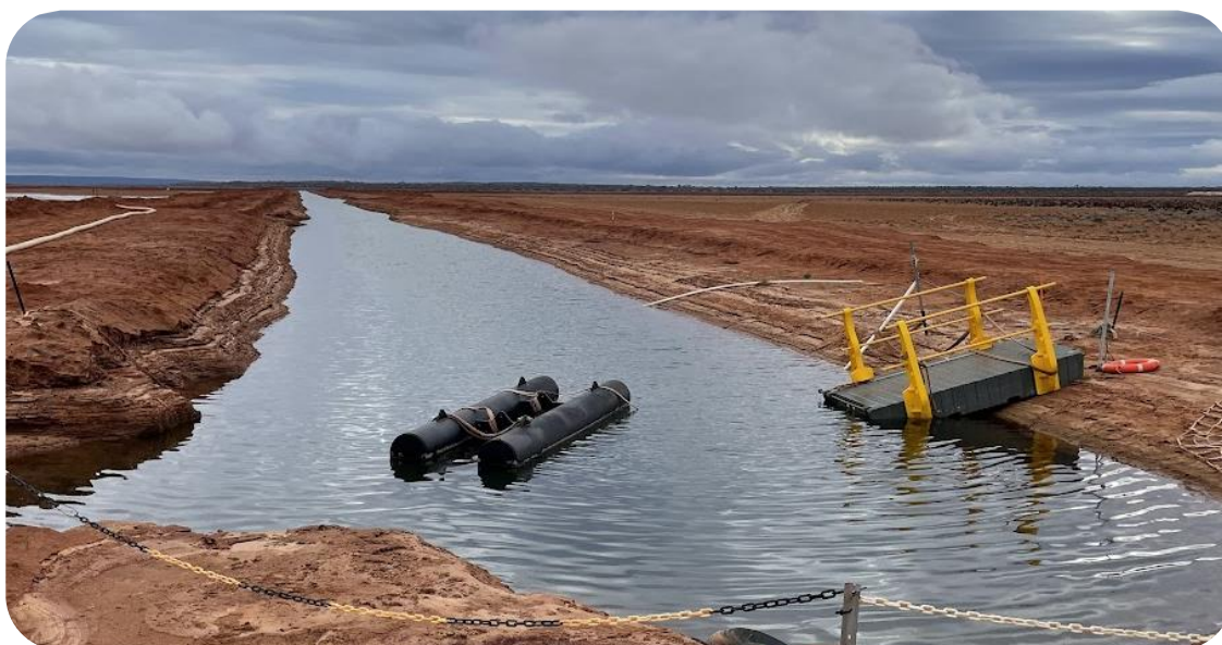
Ten Mile Trench, June 2023
