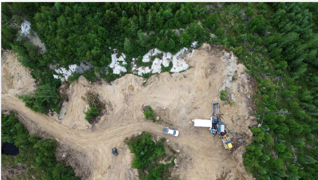
Figure 3 - Rodren Drilling at Falcon Lake
