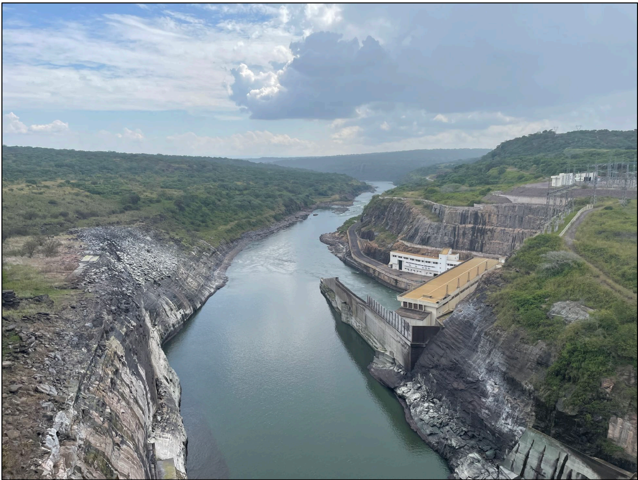
Figure 2 – Capanda Dam and Hydroelectric Facility, located in the Malanje Province of Angola.
