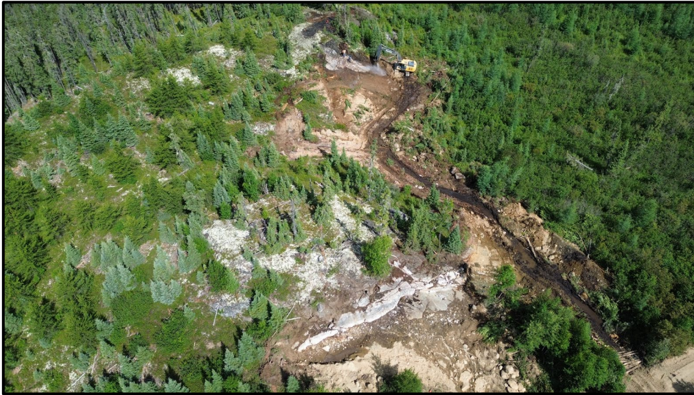
Figure 3 Mechanised Stripping & Outcrop Cleaning at Falcon Discovery in readiness for drilling.
