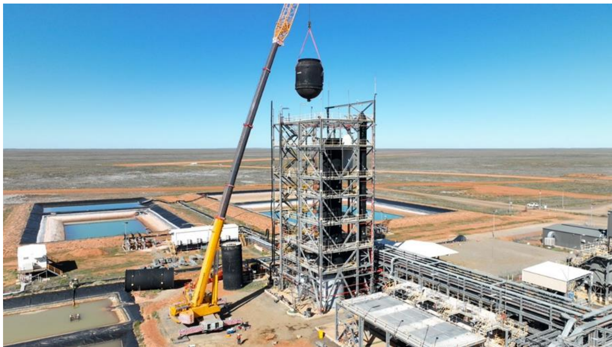
Image 3: Removal of redundant Solvent Exchange pulse columns
