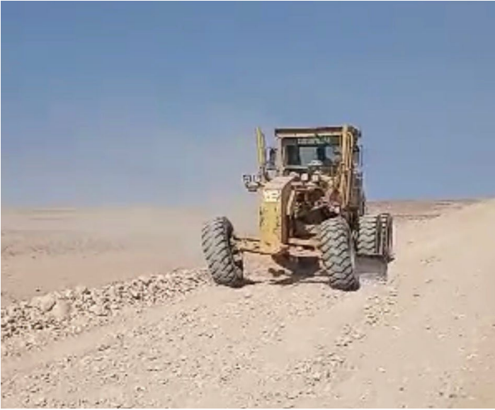
Figure 3: Work on access track improvements in-progress.
