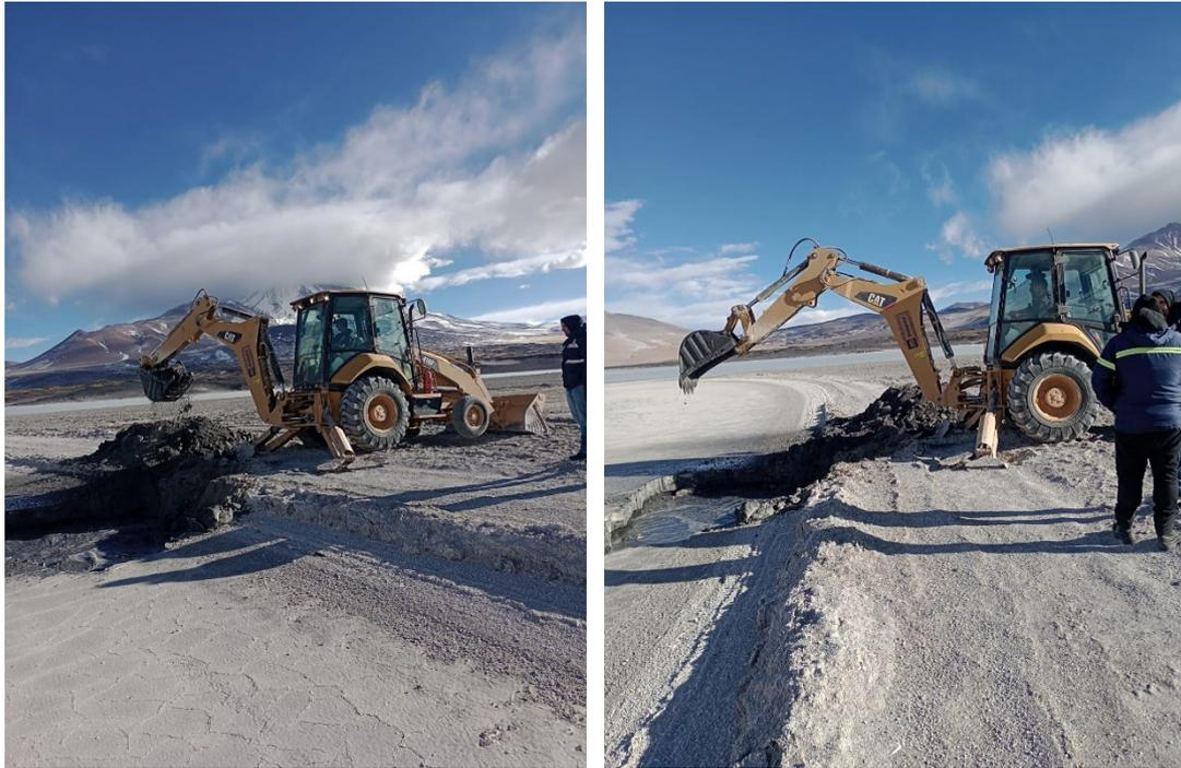
*Figure 2 Preparing drilling fluid supply for SJDD01, San Jorge Project*
