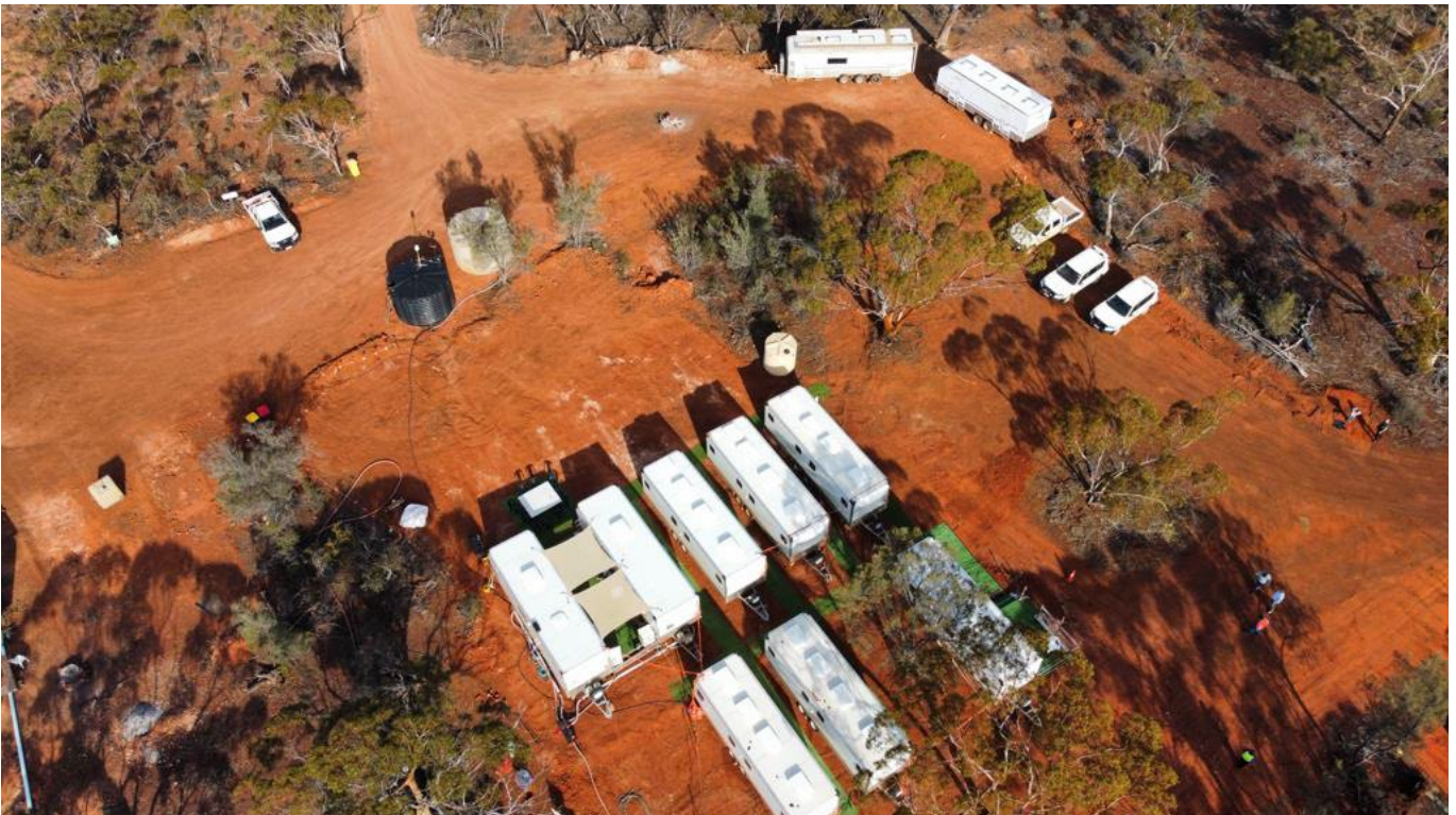
Figure 3. Expanded exploration and operational camp infrastructure at the Manna Lithium Project.
