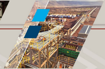
LOAD OUT INFRASTRUCTURE
