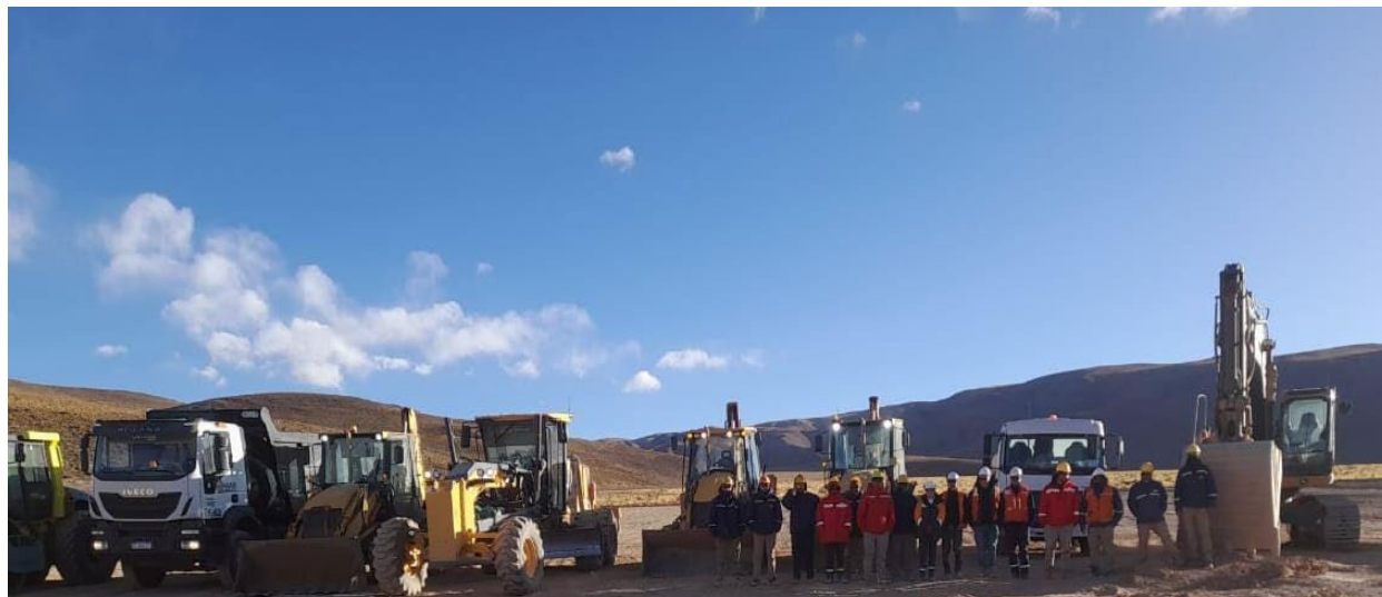
Phase 1 construction fleet and crew mobilised and on site
