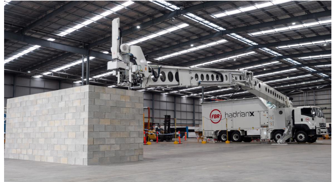
Next-generation Hadrian X® completes test build with lay-path vectoring
