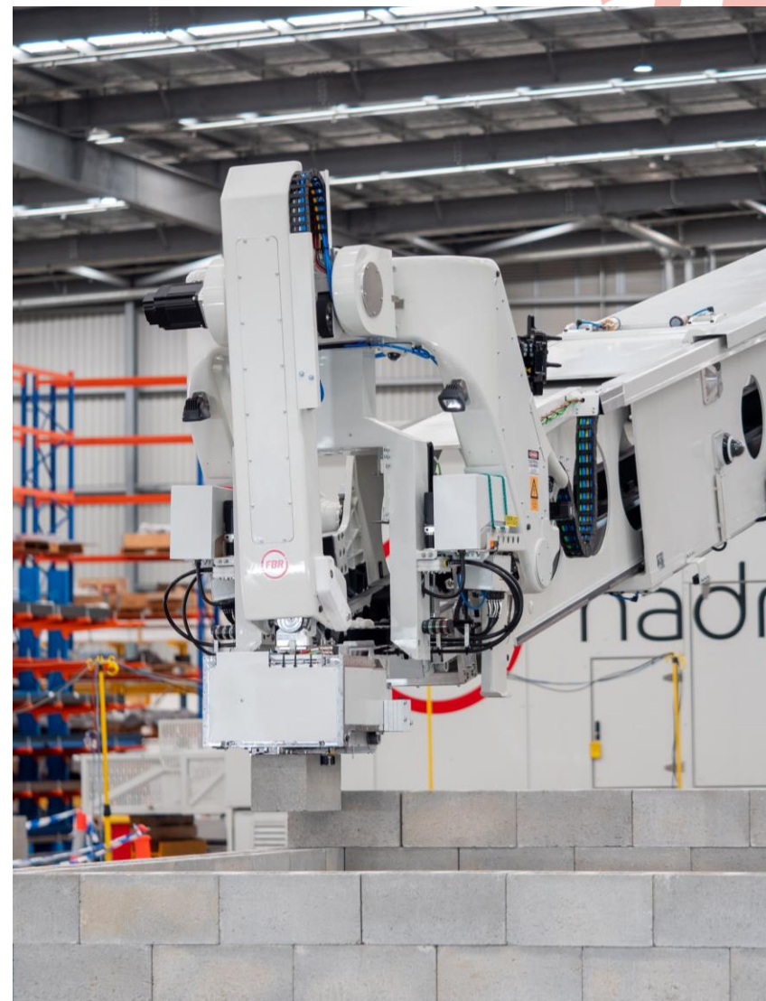
Next-generation Hadrian X ® builds test structure with lay-path vectoring
