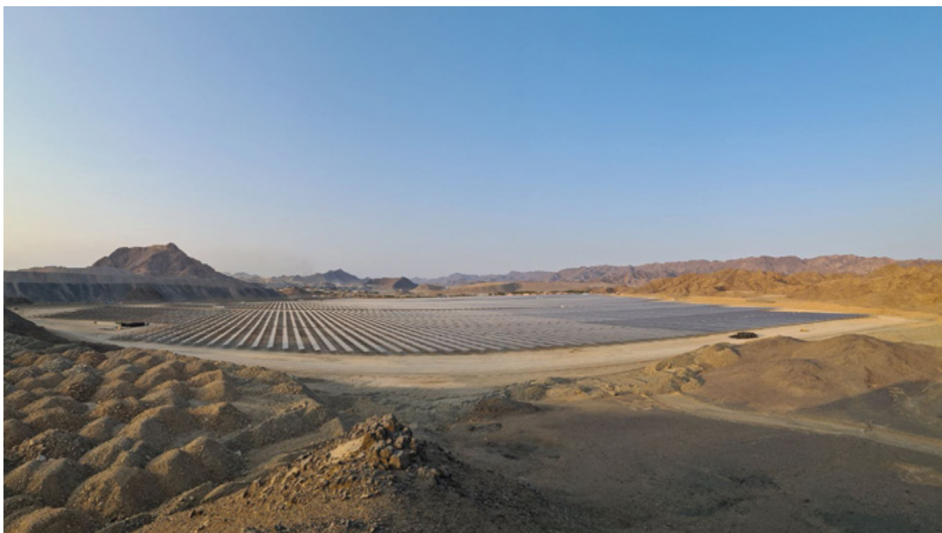
36 MW solar PV power plant, Sukari Gold Mine, Egypt
