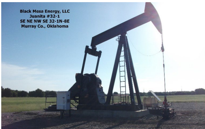
Figure 1: Pumping unit operating on the Juanita Well
