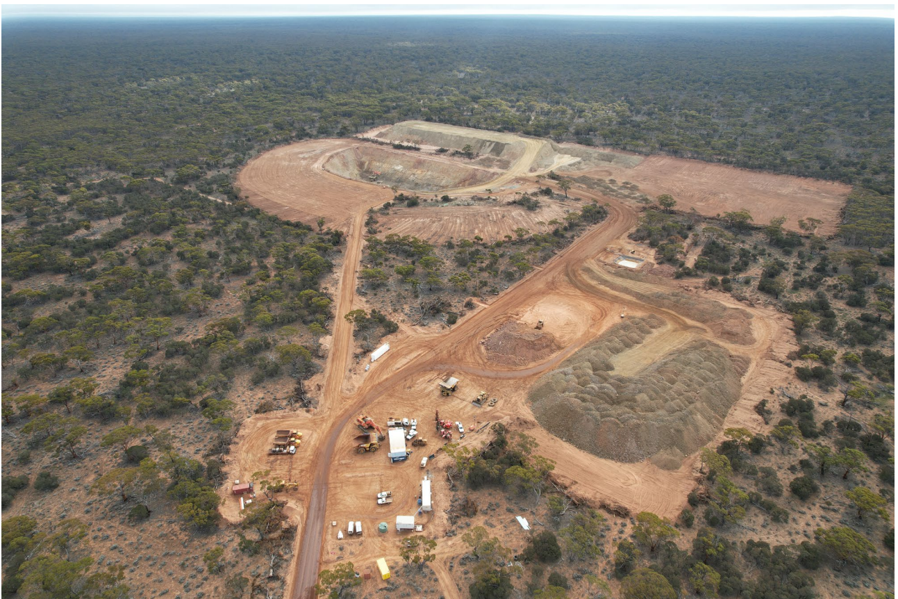
Jeffrey's Find Mine Site.
