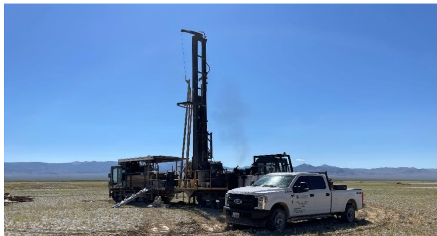
Figure 3: Sonic rig drilling at NBS Carvers
