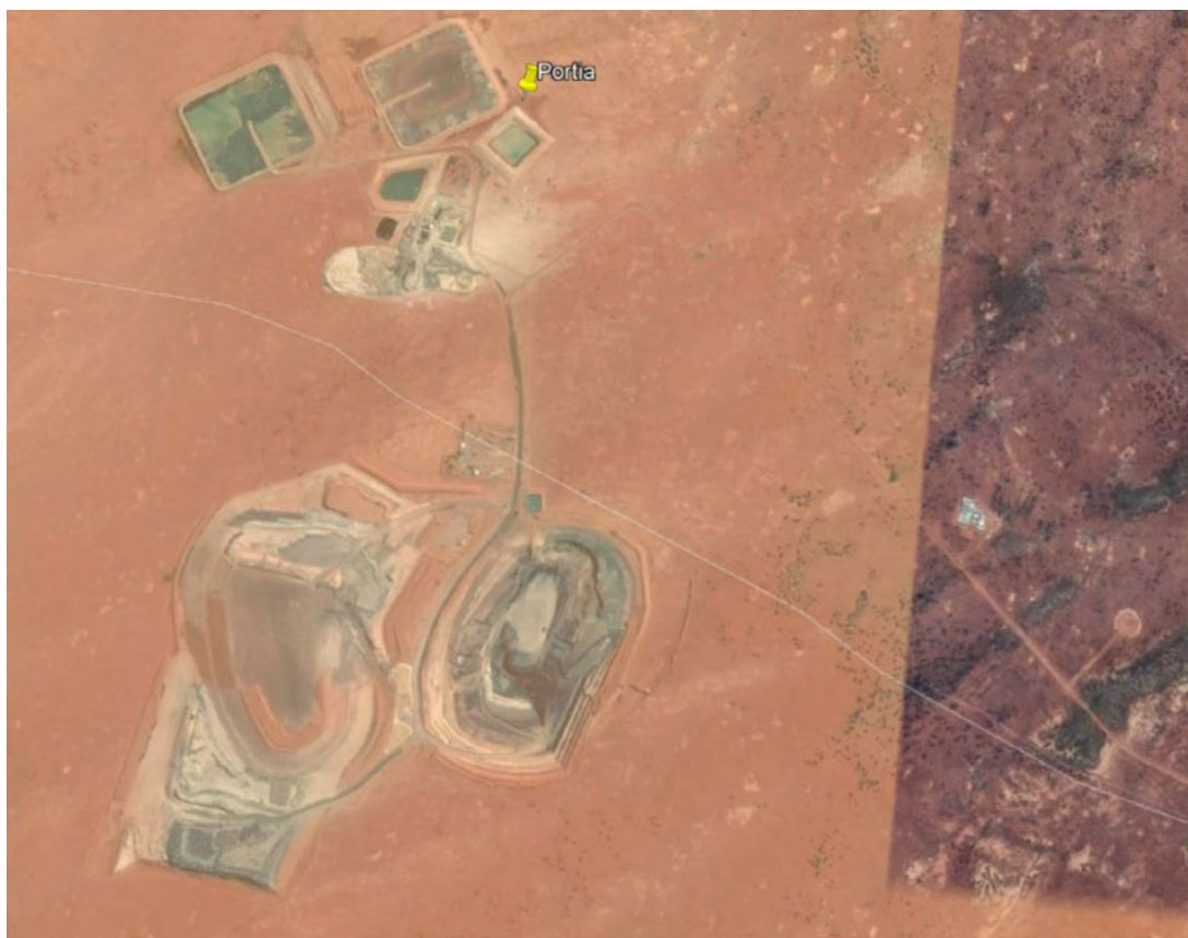
Figure 2: Portia open pit and waste dumps, with ROM pad, scrubber, processing plant (using gravity circuit) and tailings dams at the top of the image.
