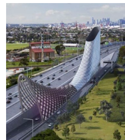
Westgate Tunnel Switchboards – Trivantage Manufacturing Over $10m
