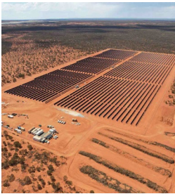
BHP Juwi Northern Goldfields Solar Project – SCEE Electrical Over $15m
