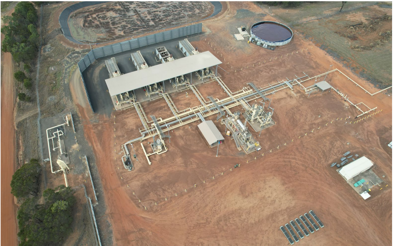
Figure: Moranbah Gas Processing Facility
