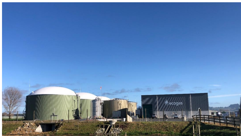
Image 2: Ecogas bioenergy facility
