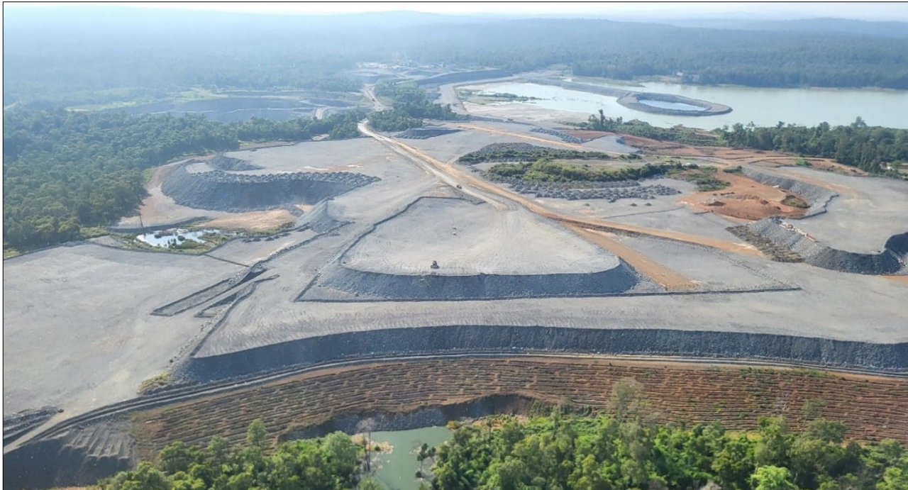
Figure 28 | Okvau’s tailings dam and waste dumps
