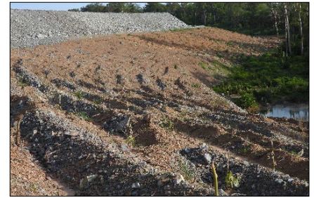
Figure 34 | Rehabilitated batter on waste dump
