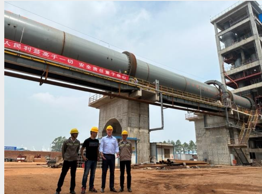
Leo and Ganfeng reps inspecting Ganfeng's new lithium hydroxide converter at Fengcheng, Jiangxi in May 2023
