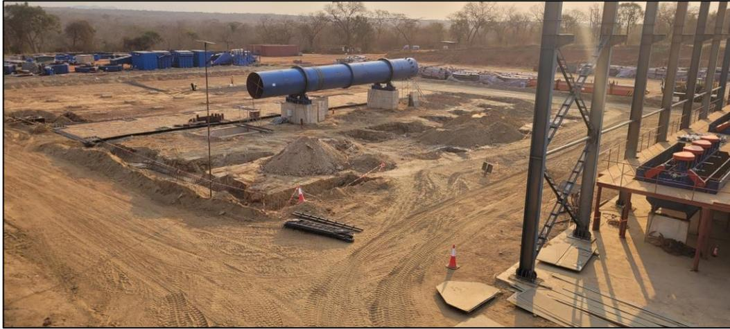
*Figure 3: Lift of the first section of the rotary dryer (top) and the complete dryer in place (bottom).*
