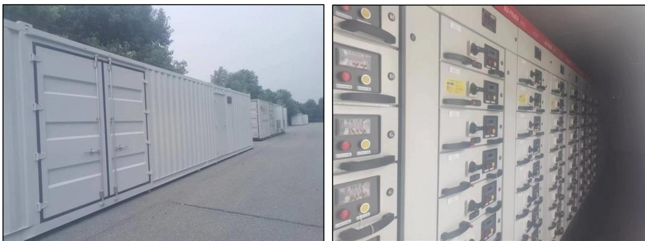
*Figure 1: Lindi Jumbo MCC's (left) and switchgear (right) upon completion in China.*
