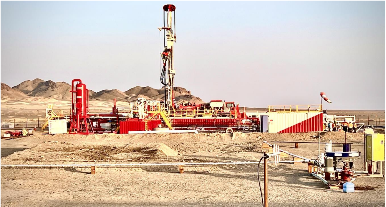
Drilling Rig at Nomgon-10
