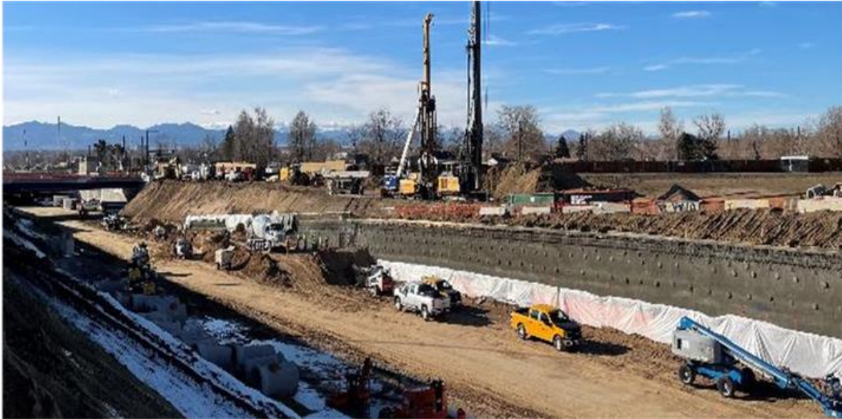
I-70 Shotcrete project in Denver
