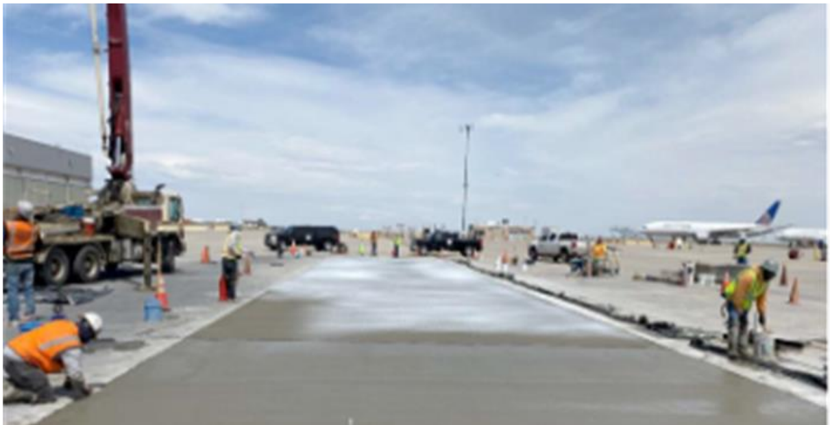
Denver Airport- concrete replacement -United Airlines
