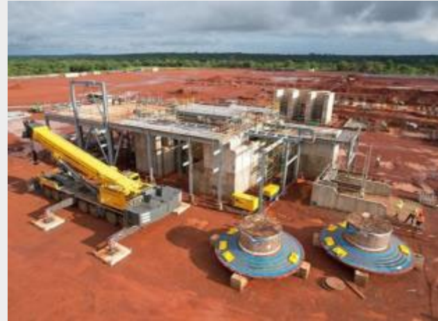
450 t crane in position for mill installation
