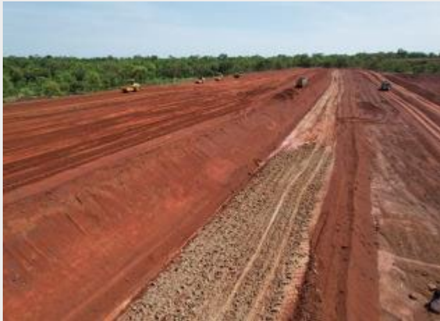
TSF embankment construction
