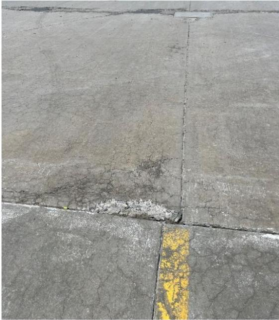
Figure 3. Section of worn concrete
