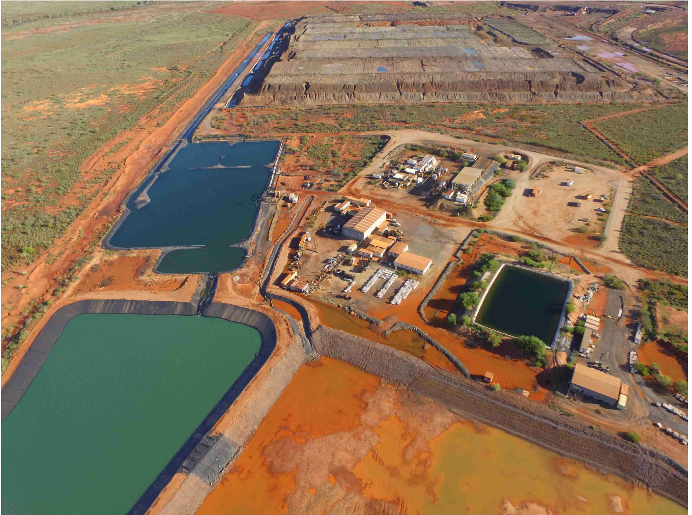
Figure 1: Whim Creek Heap Leach and Associated Infrastructure
