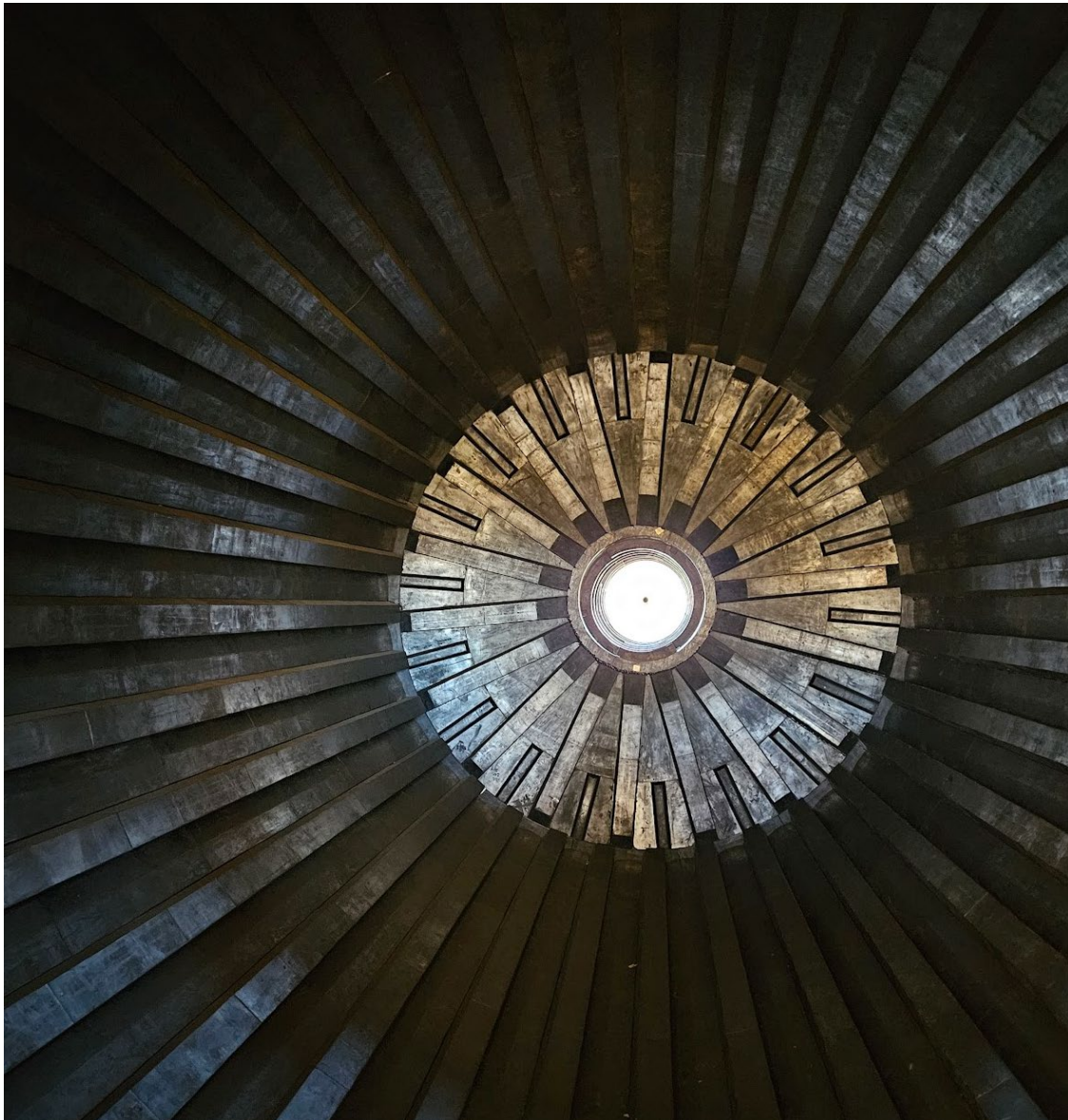
Figure 5: Ball mill liner installation complete.
